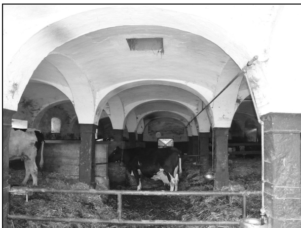
Obokana notranjost starega hleva (foto: V. Hazler, 2009).
